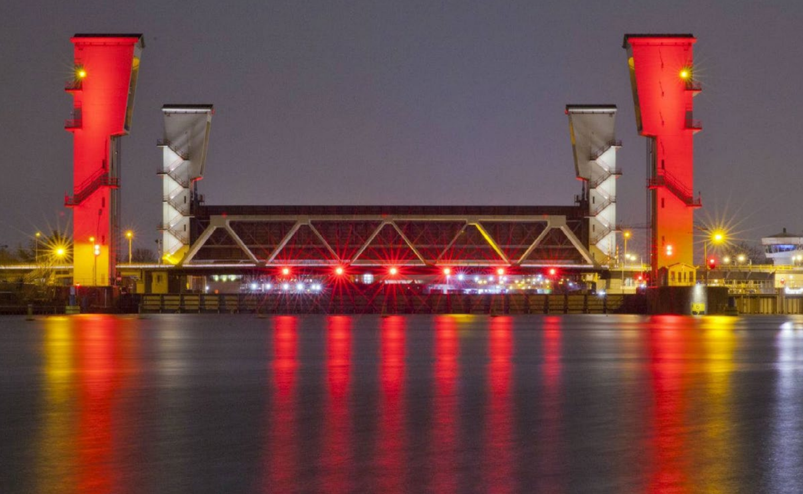
Figure 6: One of the doors of the Hollandsche IJssel Storm Surge Barrier is closing due to a storm surge at sea
