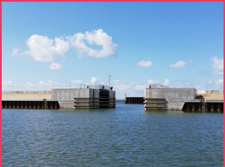
Figure 7. Example of a protection along a quay to the left (inner protection) and a barrier with a sluice gate in Esbjerg to the right (outer protection).
