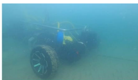
FIGURE 39 JETTING FOR THE SKAGENFIBER PROJECT.
