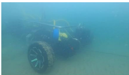
FIGURE 39 JETTING FOR THE SKAGENFIBER PROJECT.
