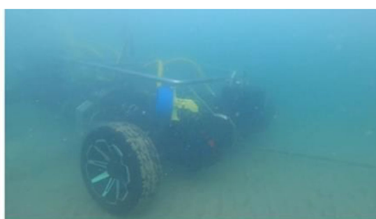
FIGURE 39 JETTING FOR THE SKAGENFIBER PROJECT.
