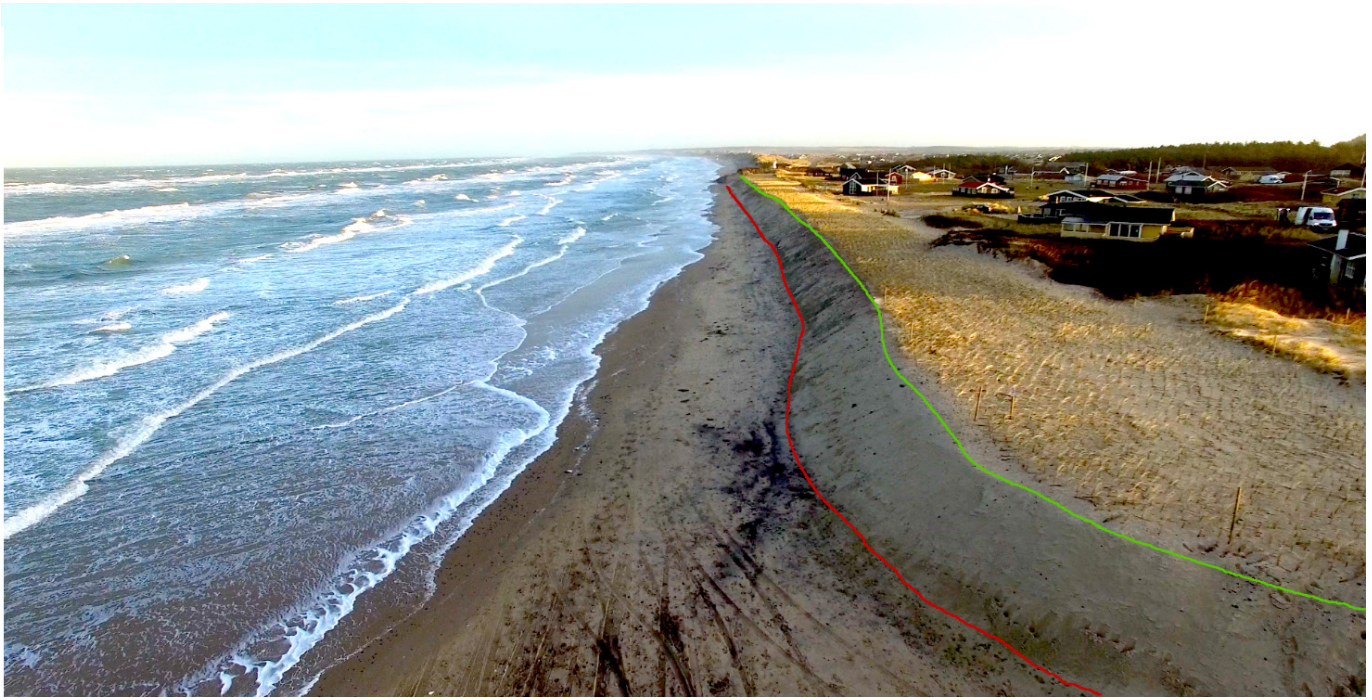
Figure 5.2 - Same as Figure 4.1, but here direction of sight is SW. The installation of the nourishment was finished on the 21-11-2016, and was measured on the 22-11-2016.
