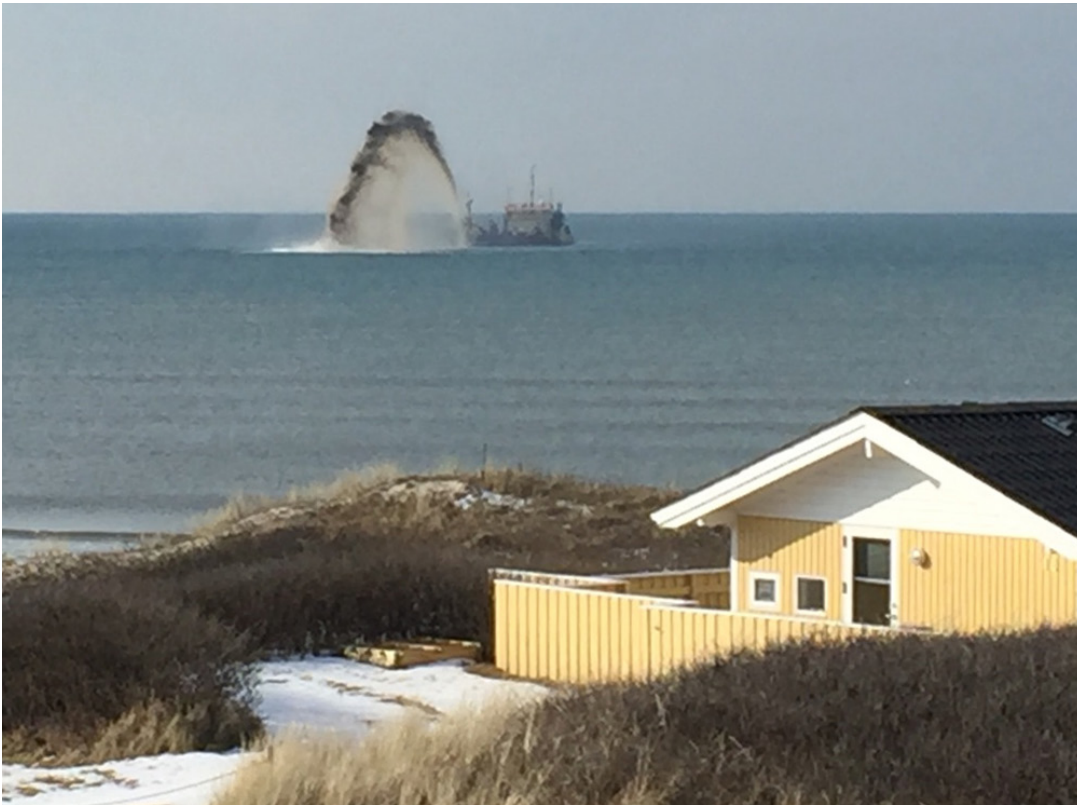
Figure 5.1: Shoreface nourishment on the shoreface outside of Skallerup Klit. No precise location of the nourishment exist.
