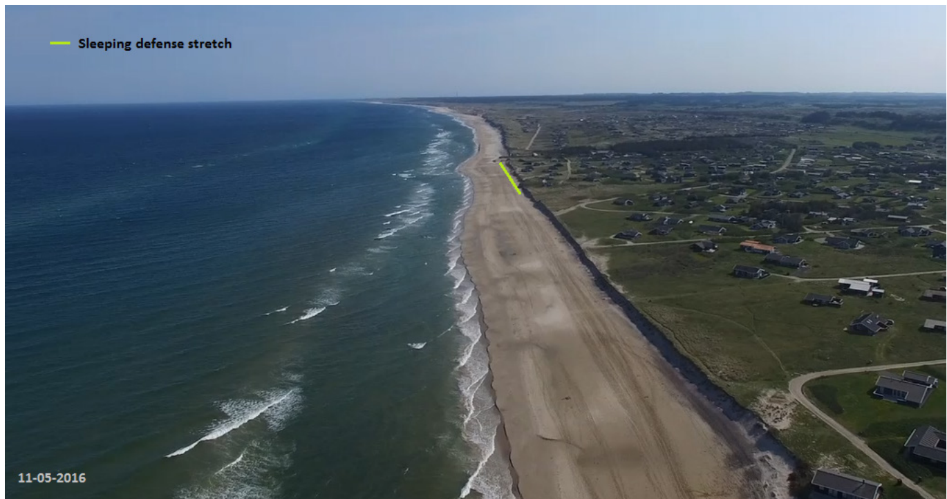
Figure 2.4: Photo is taken from “Morgenvvej” with direction of sight towards NE. The photo is from the 11th of May 2016 which is before the sleeping defense was installed. Nørlev Strandvej is located on the NE side of the sleeping defense stretch.
