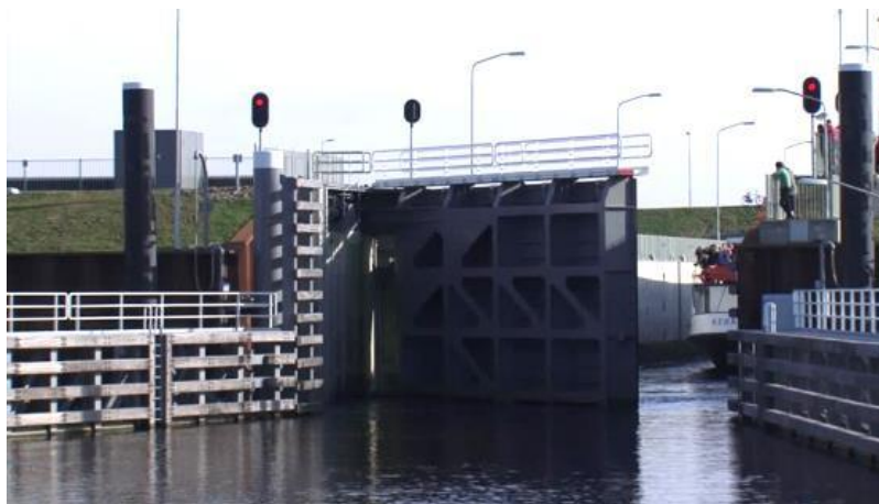
Figure 2.4 – Empel Lock, The Netherlands.
