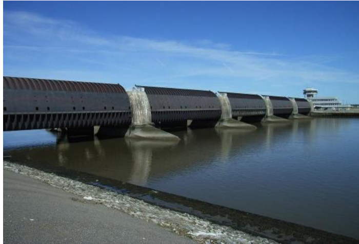
Figure 2.2 – Eider barrier, Germany.
