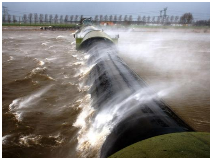
Figure 2.7 – Ramspol barrier, The Netherlands.
