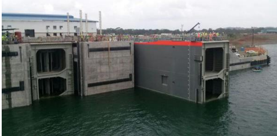
Figure 2.9 – Panama lock, Panama.
