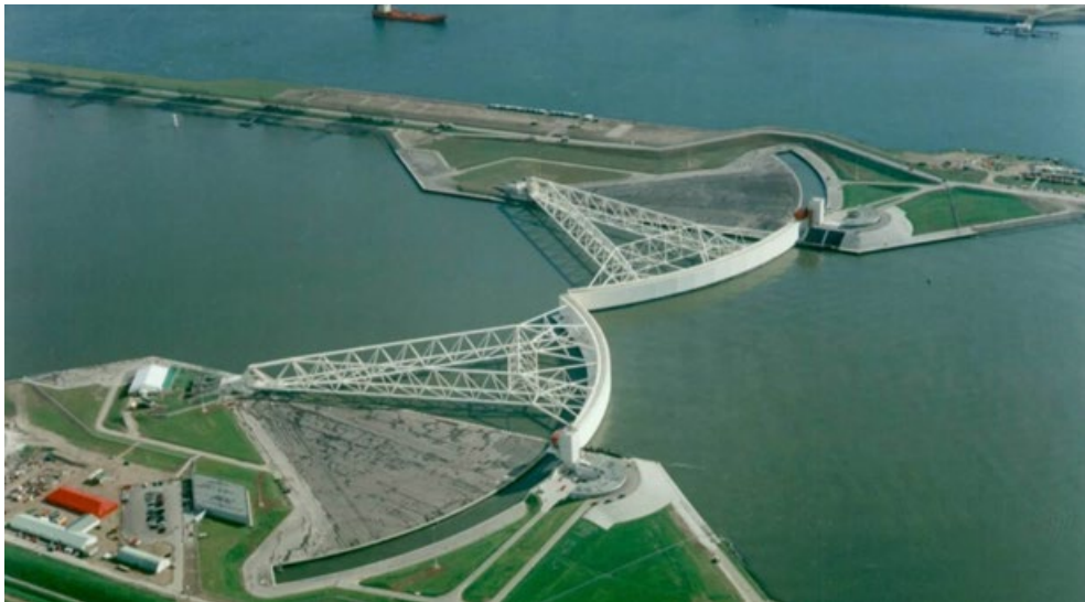
Maeslant Stormflodsbarriere, Holland (kilde: I-storm Conference 2007, Venedig)
